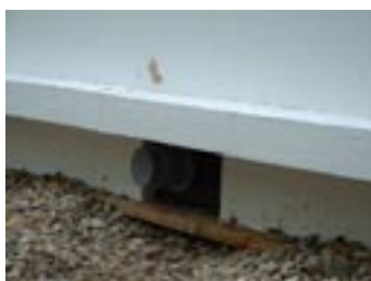
Plate 2.4 – Leachate collection drain at the bottom corner of one lysimeter
